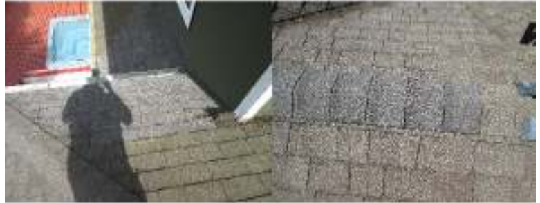
Evidence of roof repairs
